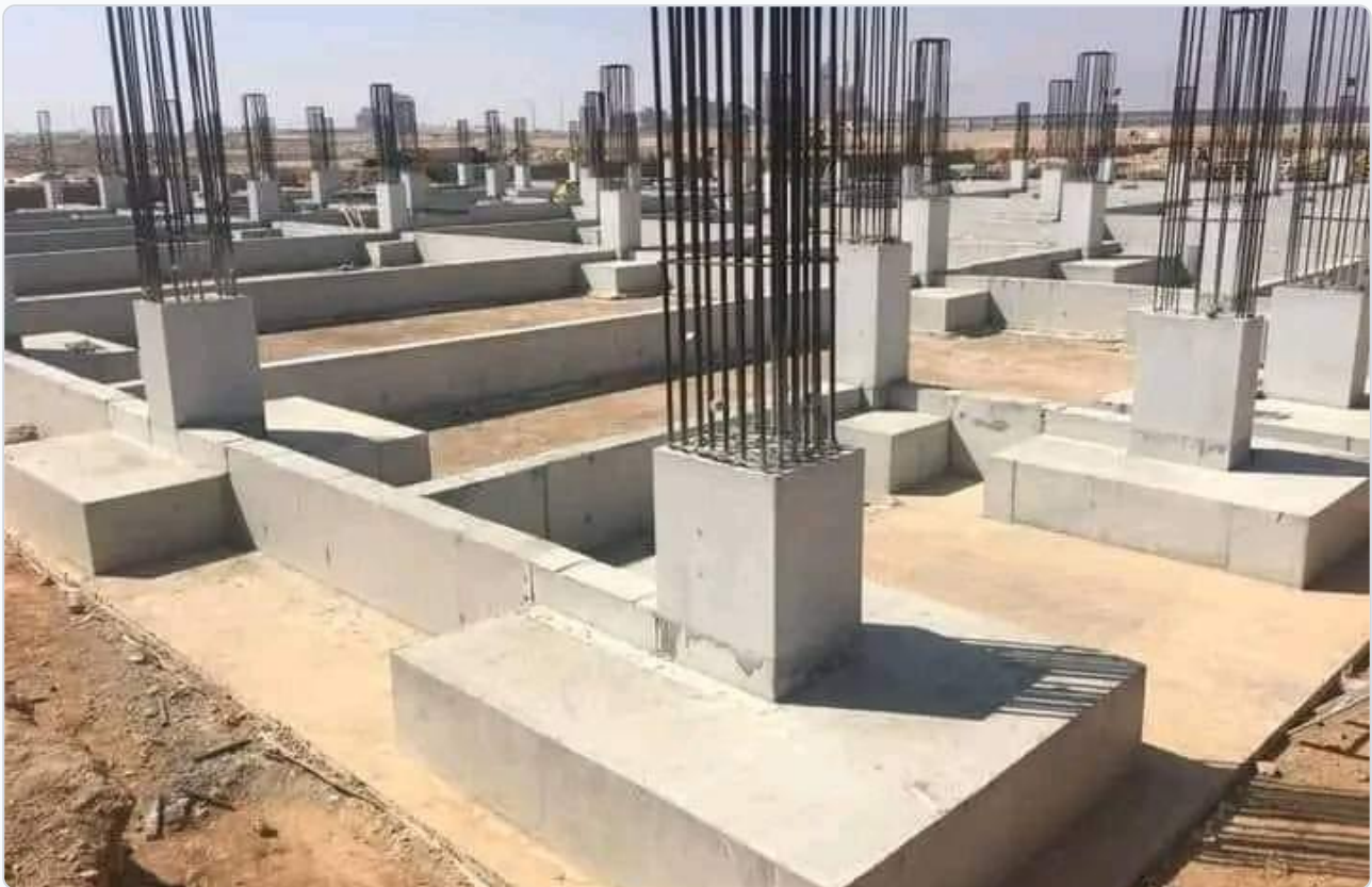
Figure 11: Heavy foundational concrete framework layouts and material staging logistics.
