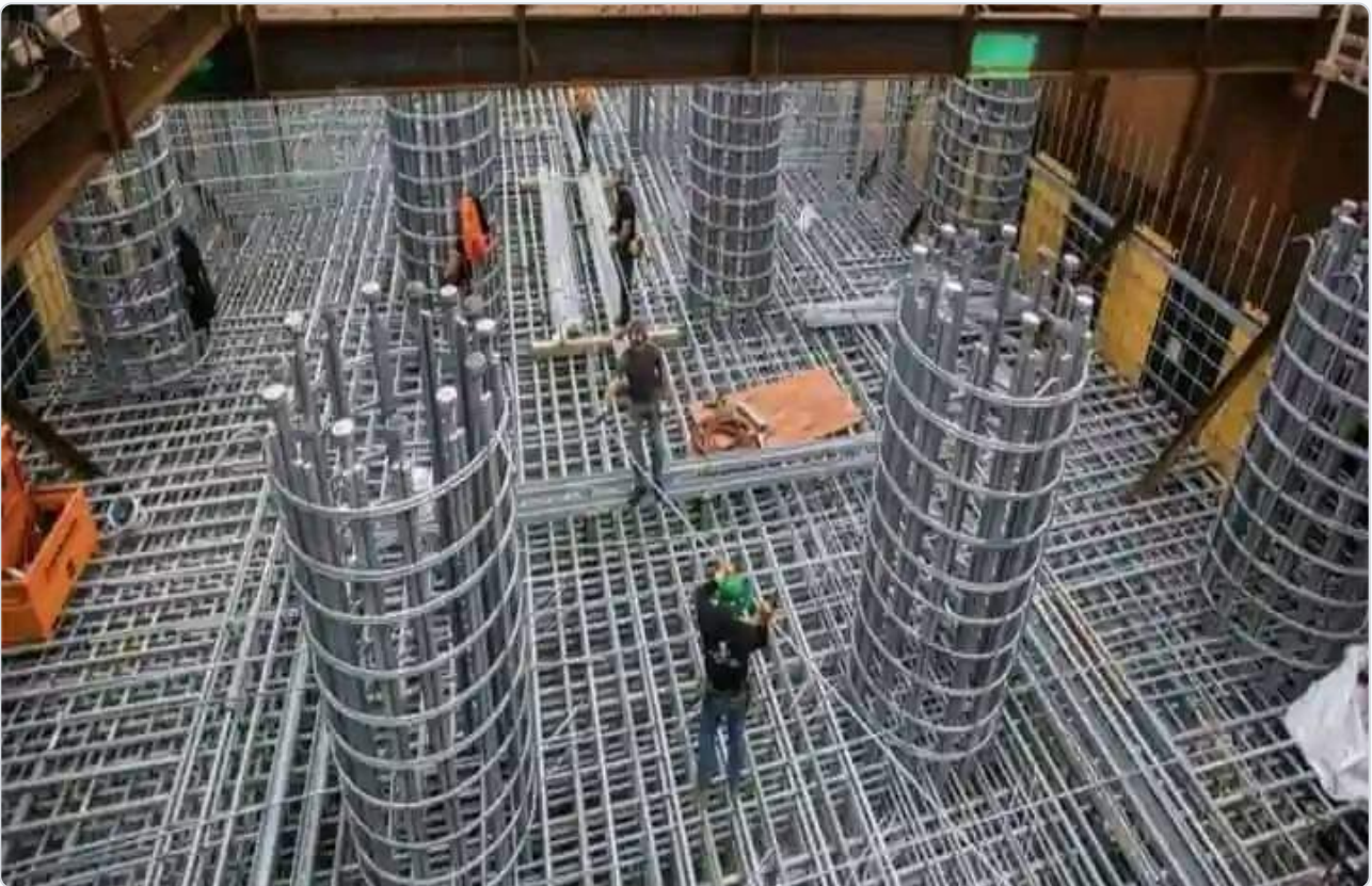
Figure 3: High-density steel reinforcement mats being placed for multi-story column frameworks.
