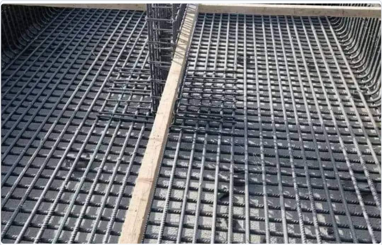
Figure 8: High-density structural slab formwork and multi-crane scheduling coordination.
