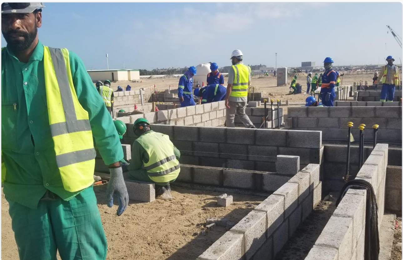
Figure 4: Direct installation of concrete block partitions by our masonry crews.
