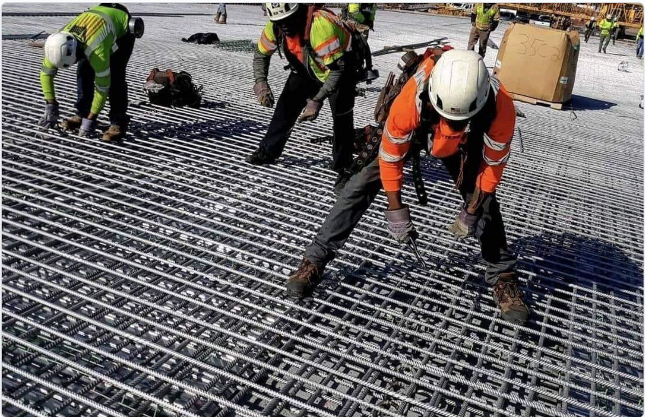
Figure 9: Heavy structural tie-beam rebar setups undergoing inspection before concrete casting.
