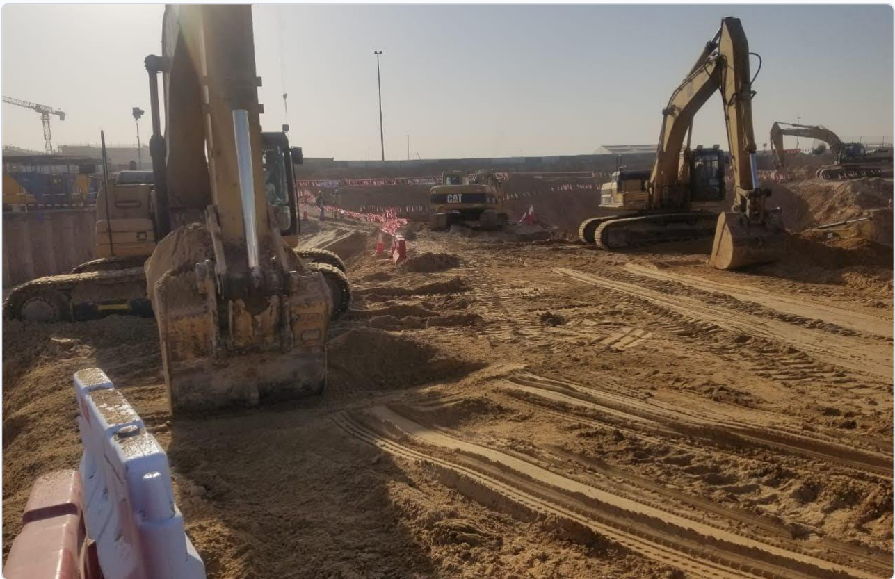
Figure 2: Mass excavation works utilizing a heavy equipment fleet and deep shoring layouts.
